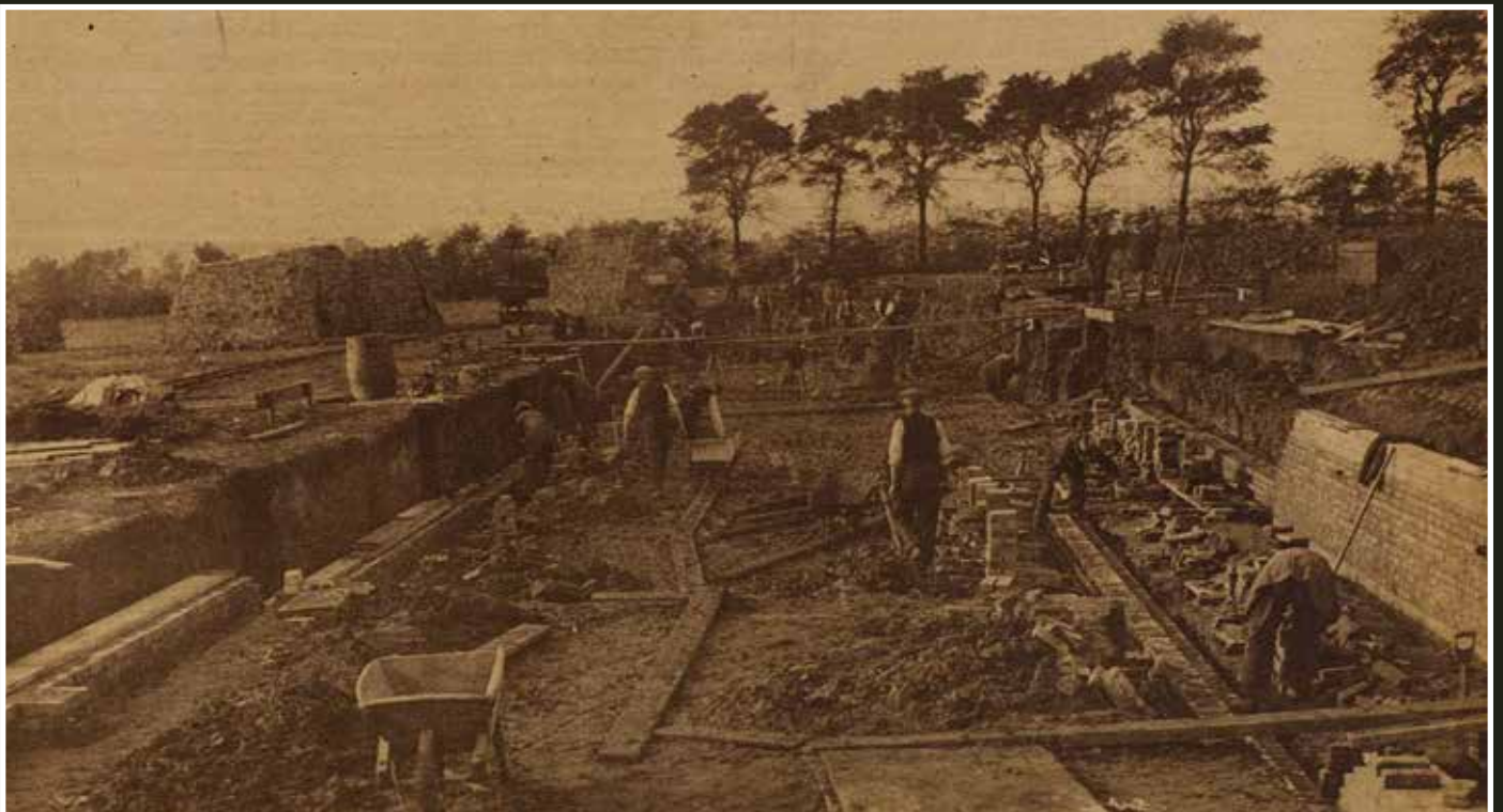
Digging the Foundations of Westcliff High School for Boys, 1924
